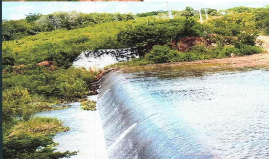
Açude Jenipapeiro II
